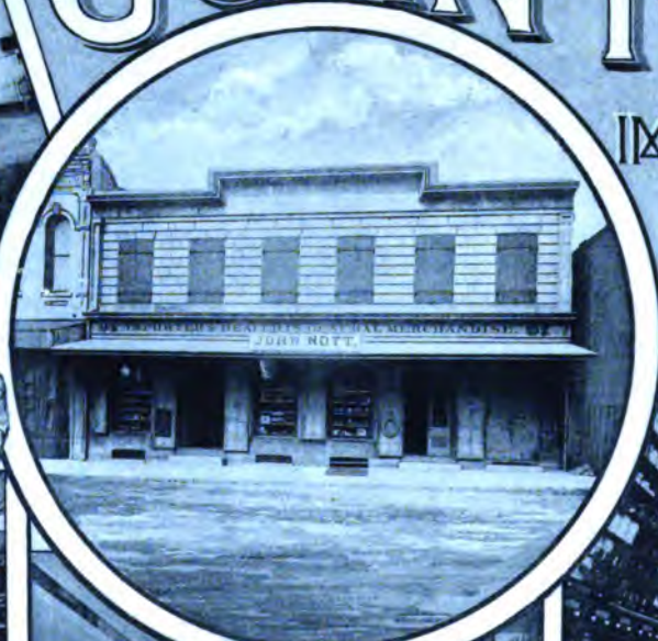
EXTERIOR OF STORE
